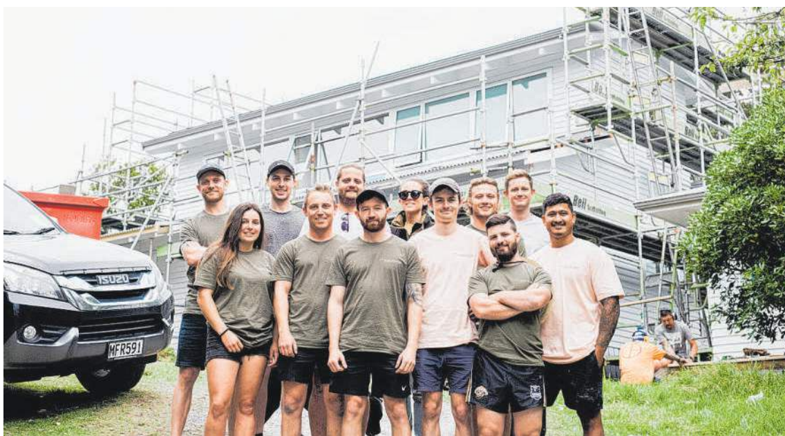
The Lightforce crew on the job at Te Whakaora Tangata's premises in South Auckland, a charity install for an organisation that works with high-risk whānau in Auckland and Northland.
